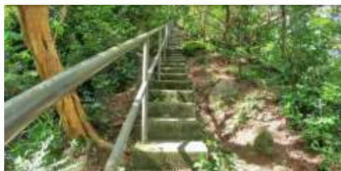
(b) Stairway crossing the berms
