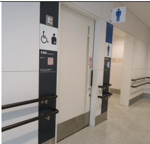
Photo 3. Power-operated sliding door
