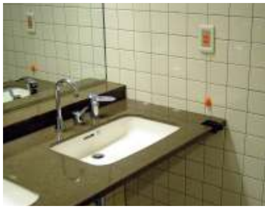
Photo 15. Basin counter edge with a notch
