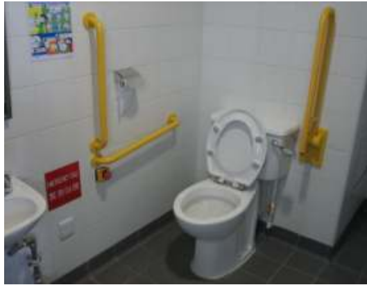
Photo 13. Grab rails in colour contrast against the background finishes
