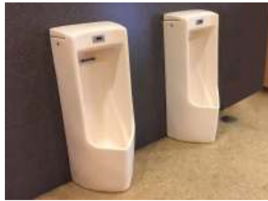
Photo 14. Sanitary fittings in colour contrast against the adjoining finishes
