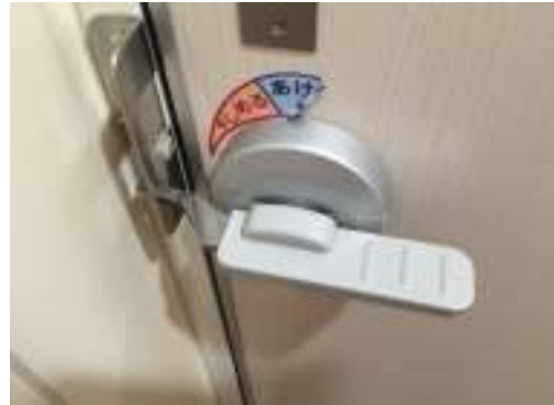
Photo 12. Easy to operate cubicle lock for sliding door
