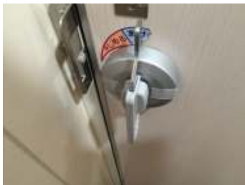
Photo 11. Easy to operate cubicle lock for sliding door
